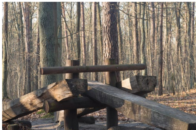
Timber from site - Larch and ash, using traditional carpentry and joinery techniques
