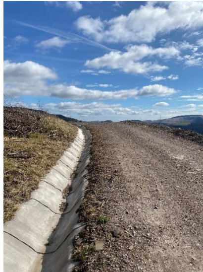
Figure 2-4: Concrete canvas lined drain adjacent to forest road
