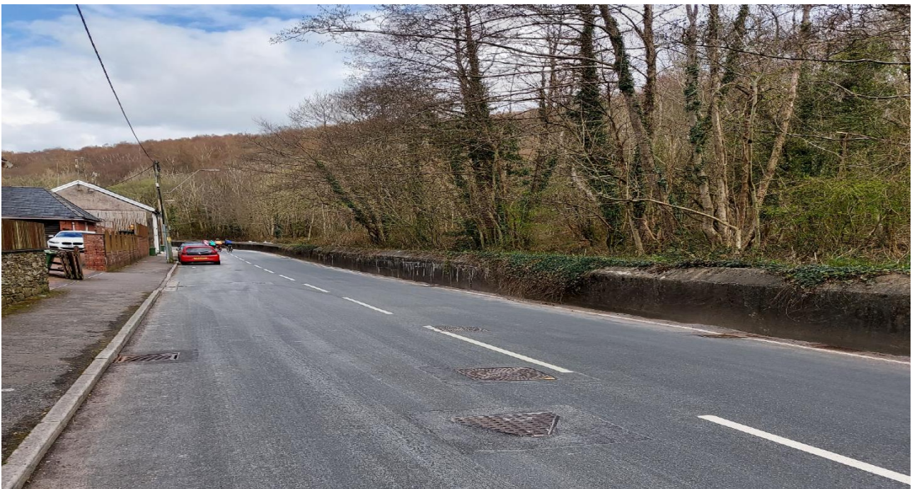
Figure 1 – Highway wall on Clydach Terrace (looking upstream)
