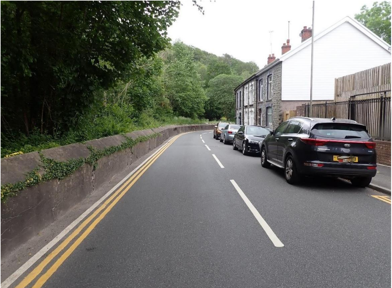
Figure 8 – Highway wall on Clydach Terrace (looking downstream)
