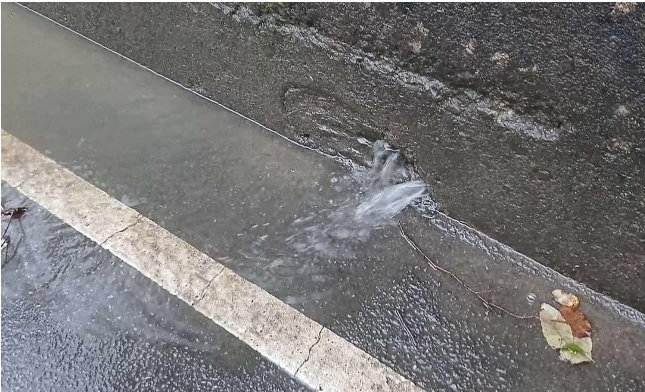
Figure 6: Water leaking through the highway wall during Storm Bert
