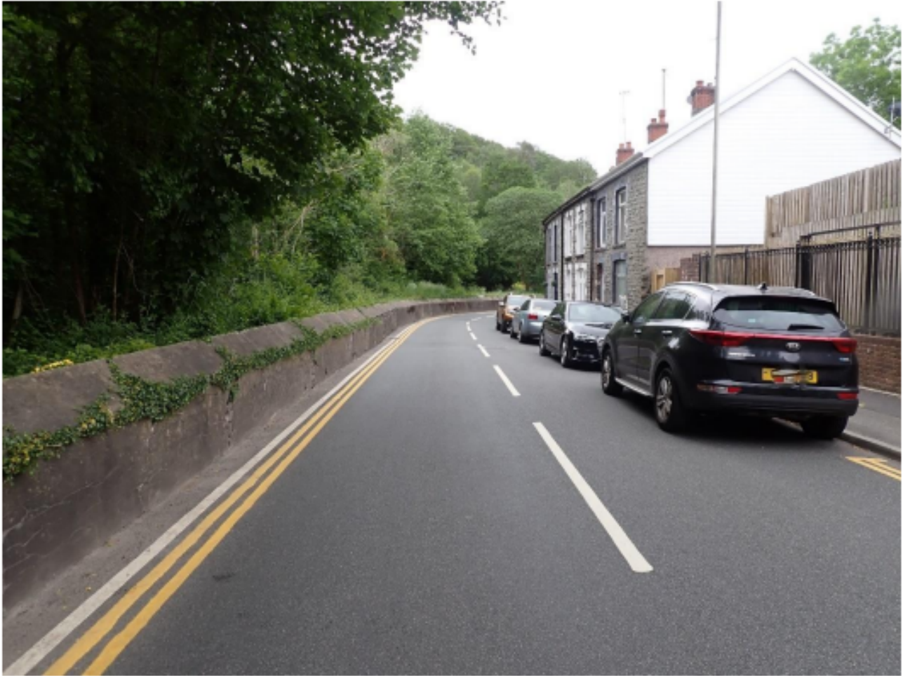
Figure 1 De-facto flood defence along Clydach Terrace (Google Streetview 2024 ©)
