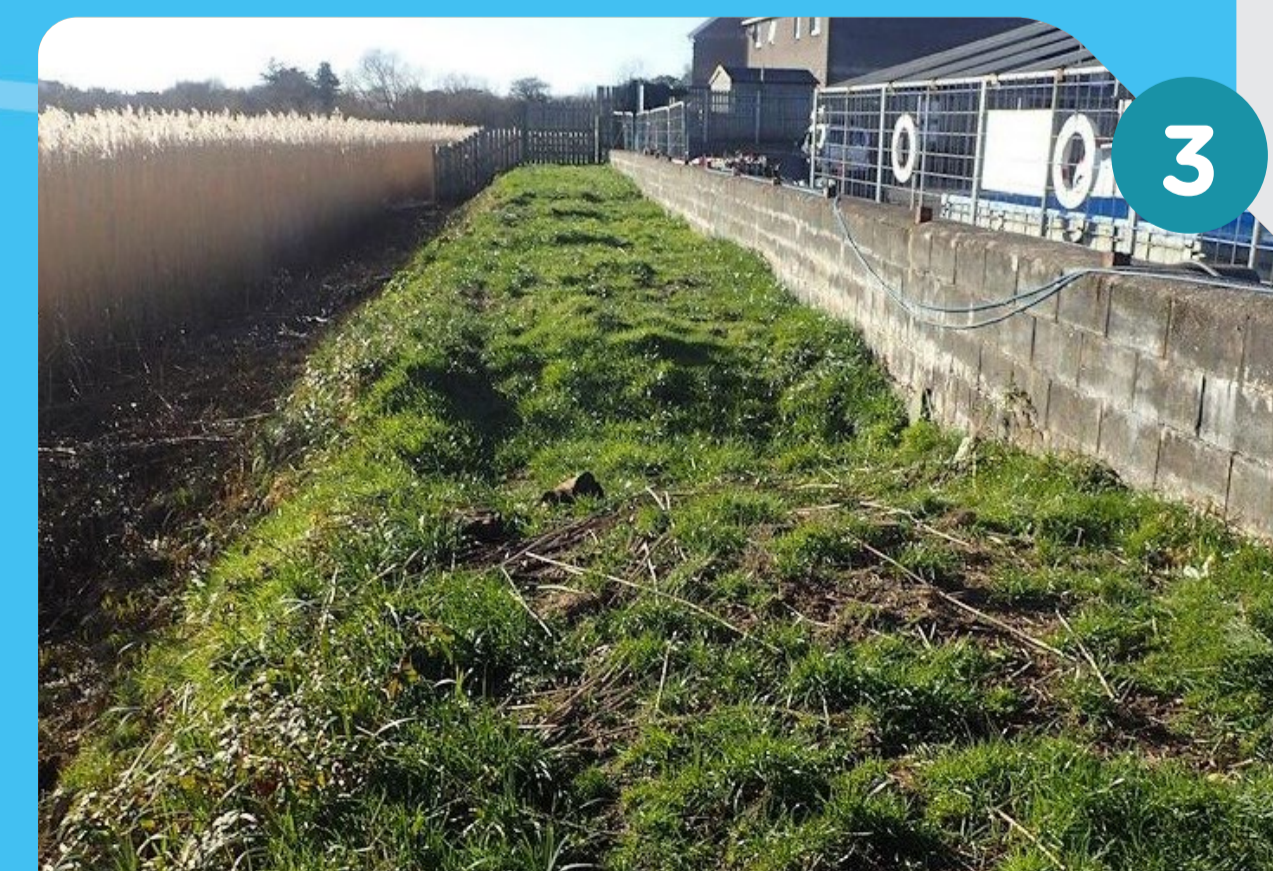
Rhyd-hir flood wall
