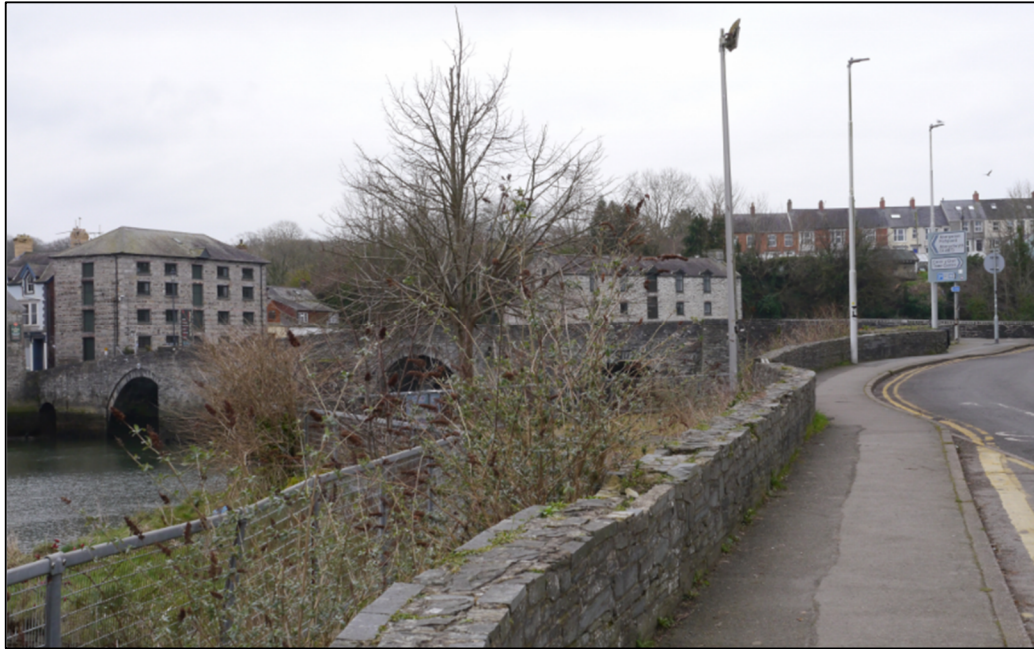
Plate 8 – Existing view of Cardigan Bridge from Strand
