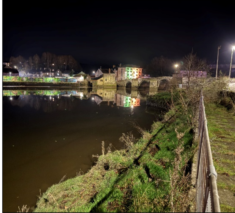
Plate 7 – Light spill onto Afon Teifi from Strand, view towards Cardigan Bridge from east
