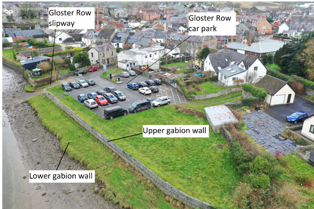
Plate 3 – Location of upper and lower gabion walls in Area 4
