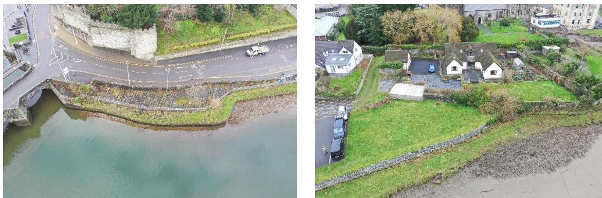
Plate 3-1 – Western extent of the Scheme (left) and Eastern extent of the Scheme (right)
