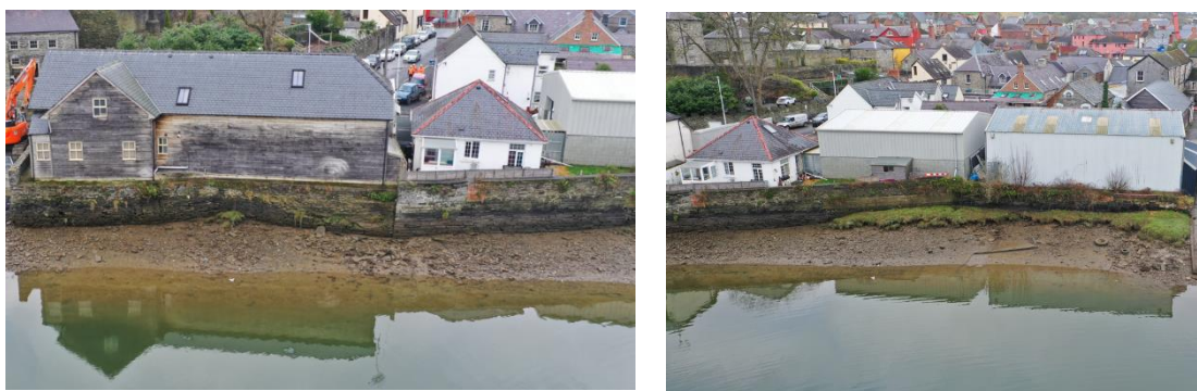
Plate 3-5 – Aerial images of Area 2
