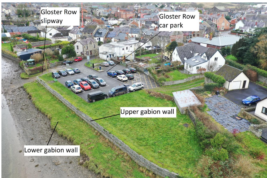
Plate 3-9 Location of upper and lower gabion walls in Area 4
