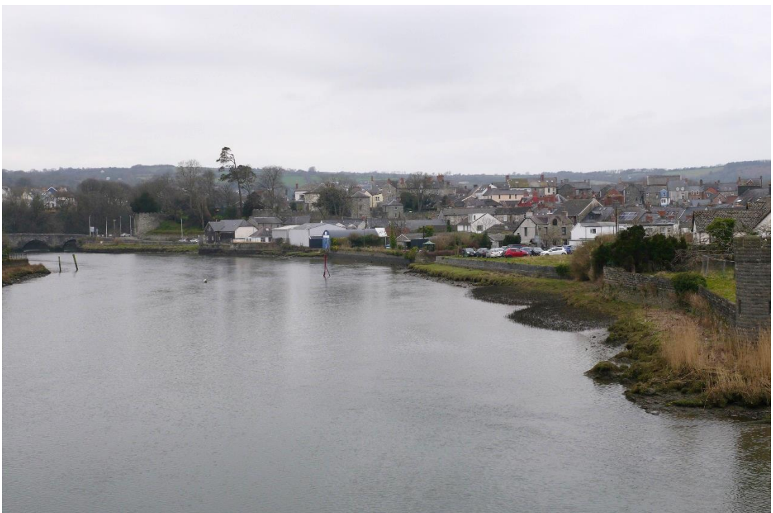
Plate 8-2: view of the north bank from Priory bridge, showing the mix of built form. Cardigan Castle and Bridge are visible downstream.
