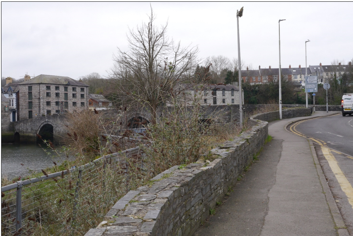
Plate 2-2: View west along Strand from the bus stop showing the riverside wall, railings and overgrown inaccessible space in between. Cardigan Bridge Scheduled Monument can be seen in the background.
