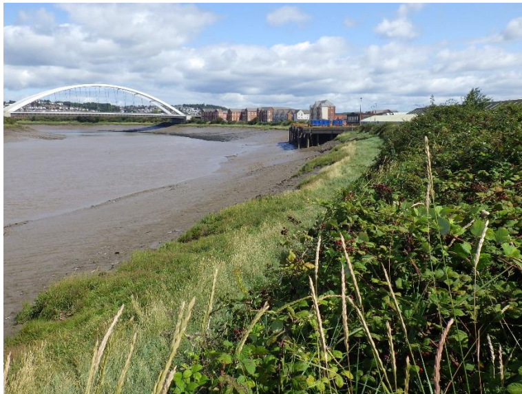
Looking north-east along the inaccessible section (TN2) towards the Orb Electrical Steels jetty.
