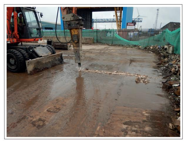
Plate 1 Working shot of 16-tonne excavator and hydraulic pecker. South facing.
