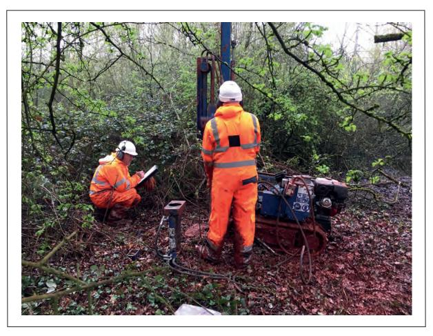
Plate 3 Working shot of dynamic probe drilling taking place. South facing.
