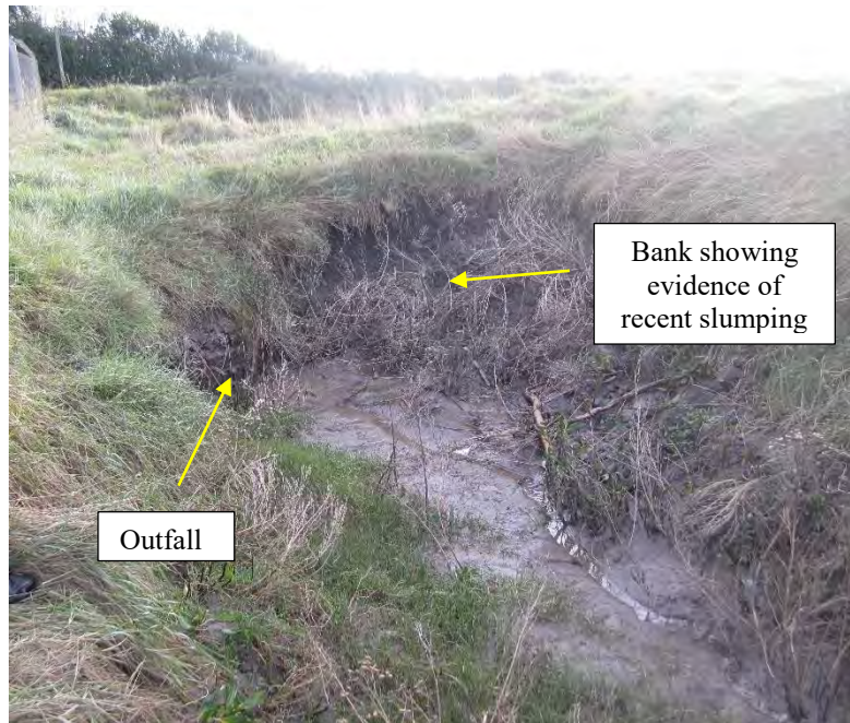
Figure 2 – Outfall 1 at northern end of embankment.
