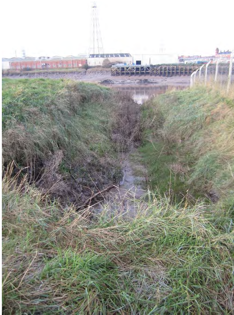
Figure 3 – Looking towards the River Usk from Outfall 1
