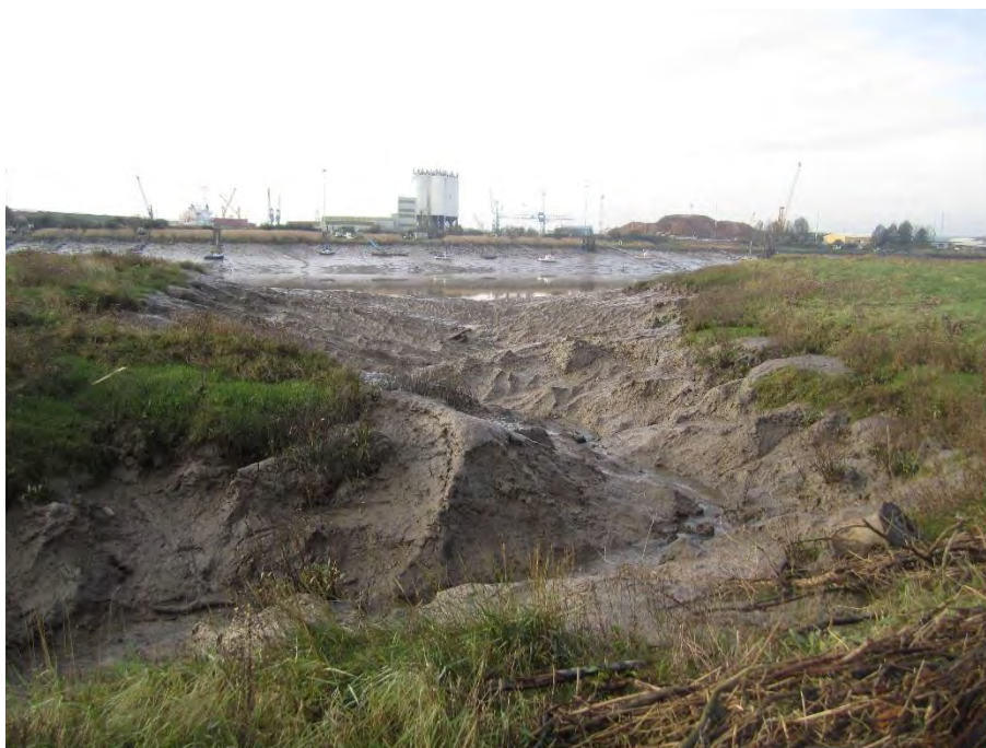
Figure 6 – Looking downstream towards the main river along the channel at Outfall 3.
